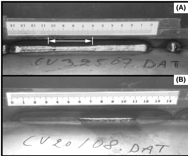
Fig. 5 — T-joint with step disturbance No. 1. Photo of: A — Front; B — rear side of a welded joint. Note that the weld joint at the front of the T-joint in the interval 6–10.5 cm, along the scale (where the weld joint tapers) deviates from normal weld quality, i.e., the size of the leg length and throat dimension is reduced.
