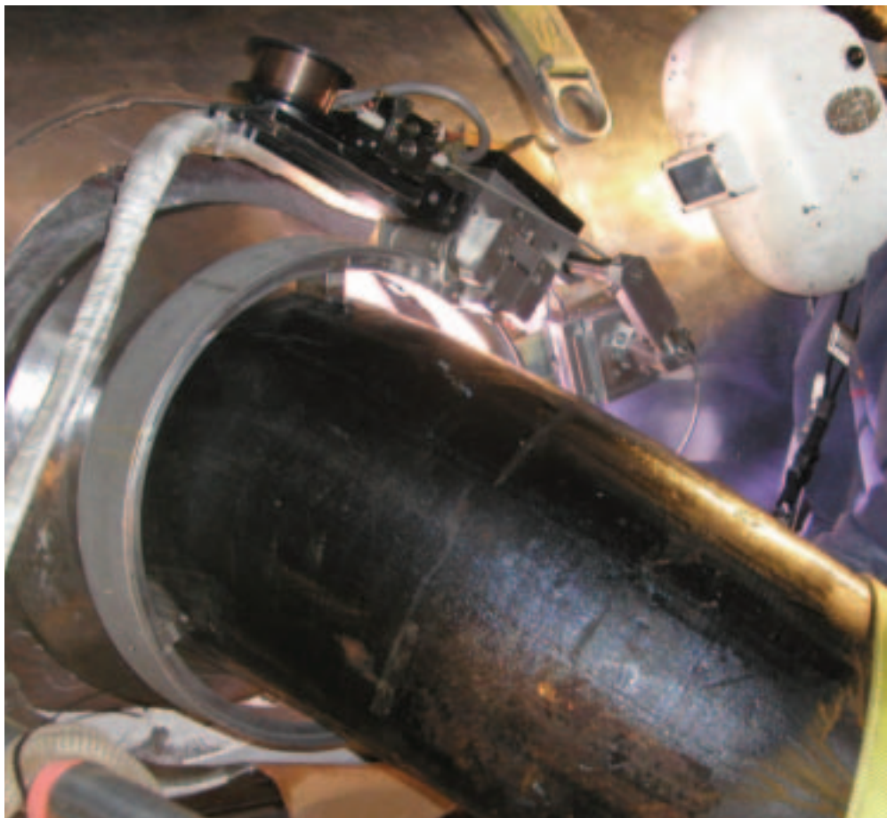
Machine gas tungsten arc welding of a pipe-to-nozzle joint.
