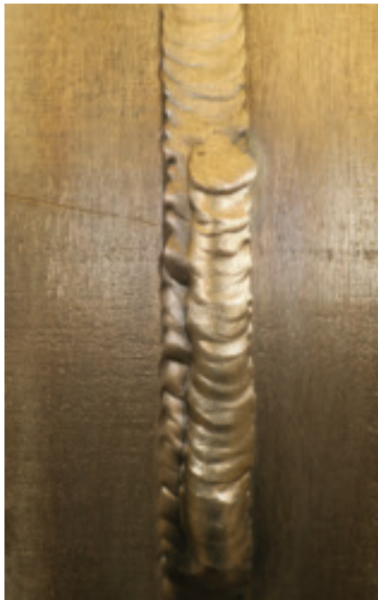
Make subsequent passes using the stringer bead technique.
