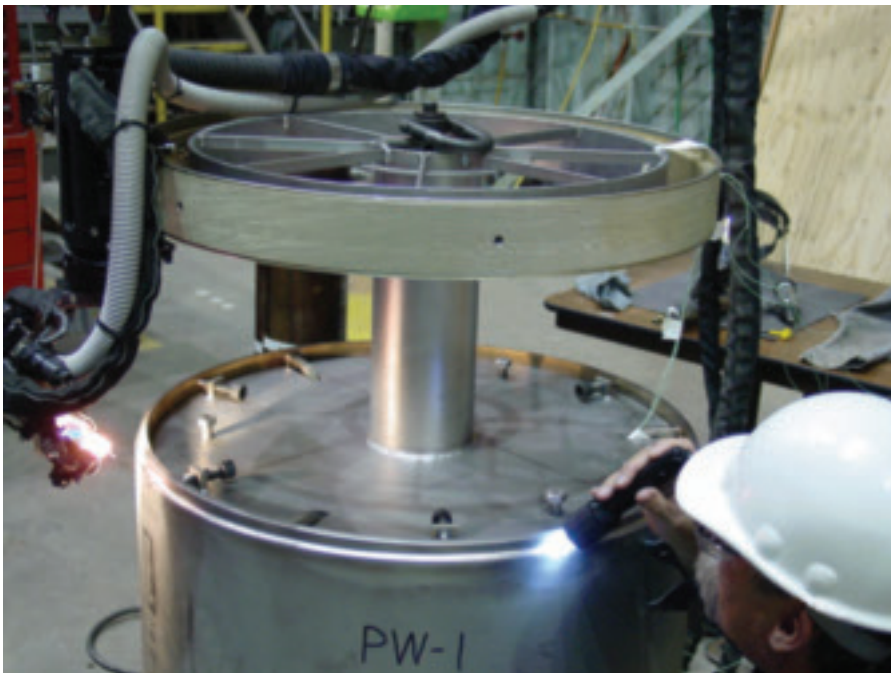
Fig. 1 — This designed and fabricated fixture supports and aligns the weld head during welding.
