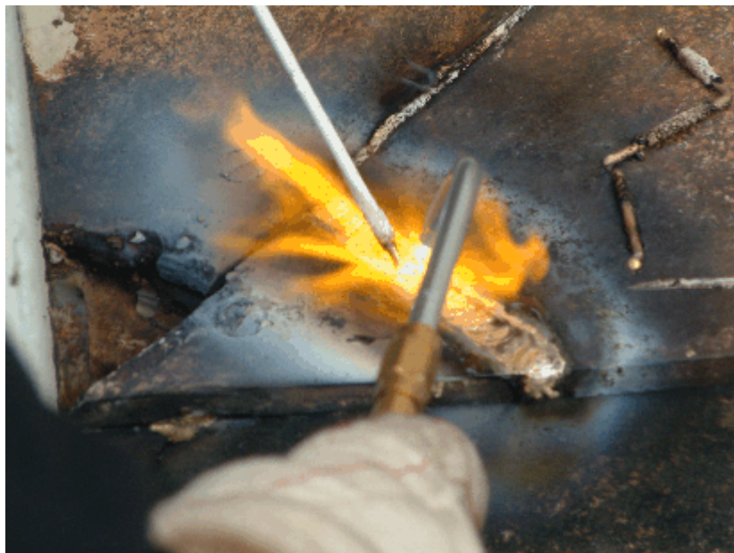
Figure 3. Location 1 - making the repair by braze welding.
