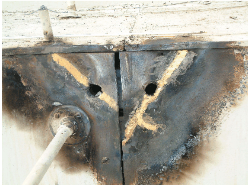
Figure 4. Location 2 - after finish grinding, but before painting.
